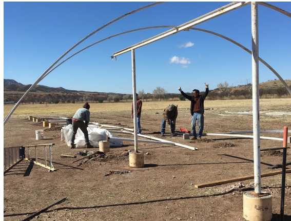
Greenhouse construction in action! [p.c.- BRN]
