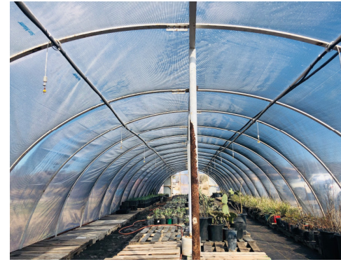
Greenhouse with permanent shade cloth and a soft plastic layer that is added or removed seasonally. First photo shows plastic on, second is with plastic off. [p.c.- BRN]
